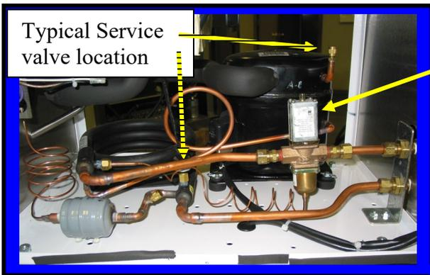
Valves automatically open on pressure increase, close on pressure decrease. **Adjustment:** To raise valve opening point, turn adjusting screw, on top of valve, counter-clockwise. To lower operating point, turn clockwise. Opening point of valve should be raised just enough to cause valve to close when compressor is off.
