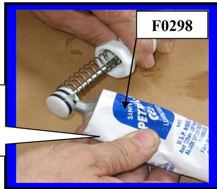
Installing **Plunger Assembly** into Faucet body
